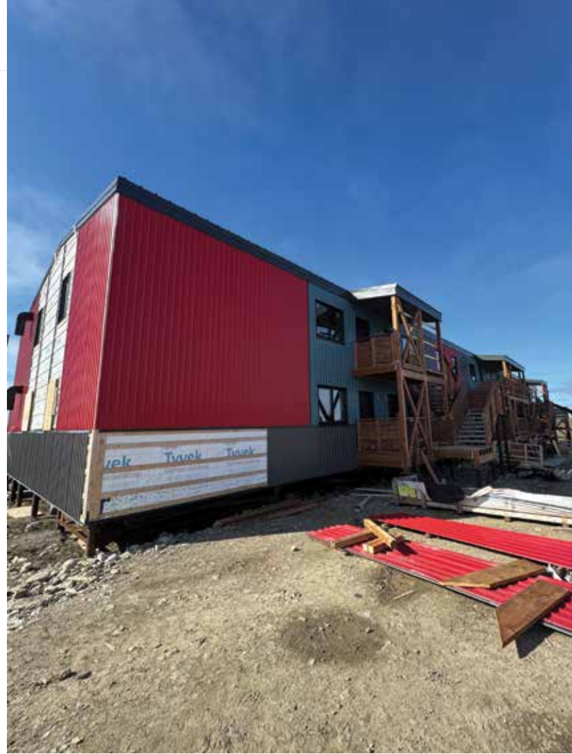
↑ ABOVE: 📍 Cambridge Bay. 12-plex under construction, July 2025.
