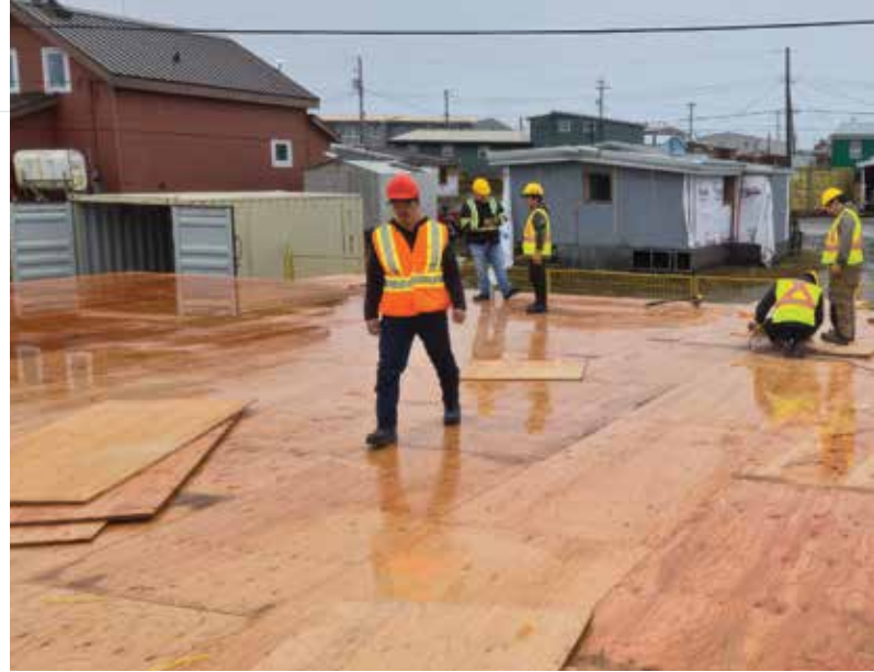
↑ ABOVE: Floor assembly underway.
